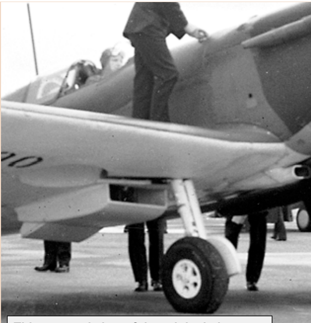
This cropped view of the original photo shows a lot of underwing detail of the 'white' side of the aircraft. Note the (mostly) white wheel well, wheel hub, undercarriage leg and door. The small black circle on the side of the cowling is for the manual engine crank handle. Below is it a small brass plaque with the ground crew warning instructions. DND Canada photo PL-371, 16 May 1940
