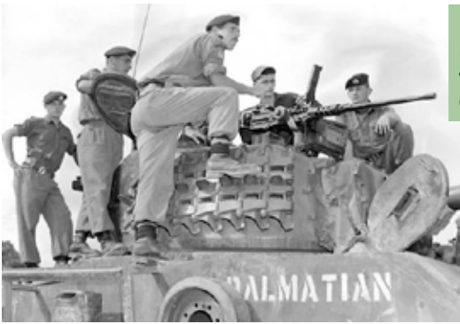
▼ Members of C Sqn bringing one of the spare Shermans forward as a replacement for a broken down or damaged tank. It has a roll of barb wire and a .303" ammunition box attached to the front fenders. A spare road wheel is mounted onto the turret side. (Library and Archives Canada PA-133619, DND photo via Anthony Sowards)
