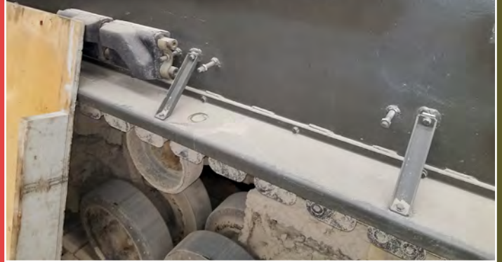
Another view of the side extensions. Also seen here are the two mounting bolts for each of the three spare track links carried on each side, along with a good view of the track retaining clips that hold them in place. Steve Sauvé photo, July 2018
