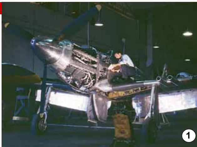
A Mustang Ia/P-51 during assembly. Please note the rear of the wheel wells are not like the "wall" of the Accurate Miniature kit, or any other Mustang kit, the main spar is the back "wall" of the well. Smithsonian Institution Image
