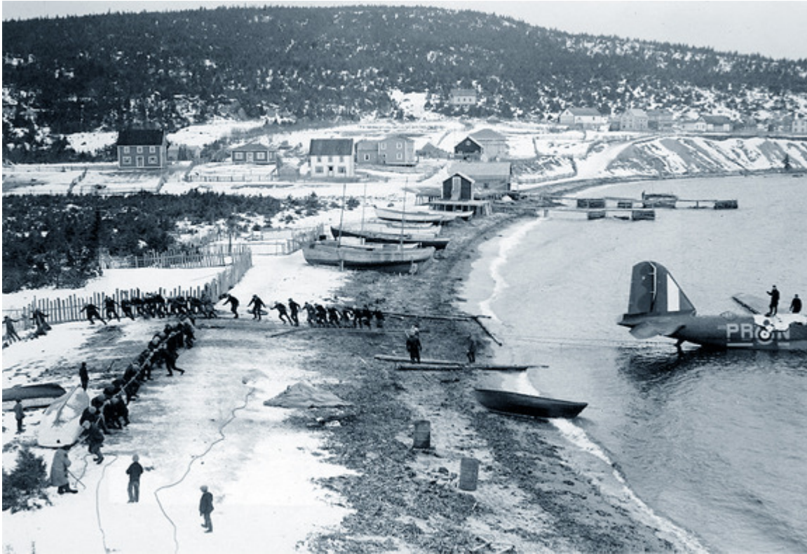
Haulin' in the Digby. Ground crewmen of 103 Squadron pull a Douglas Digby flying boat on to the beach for a barnacle inspection. Photo: The Shipping News
